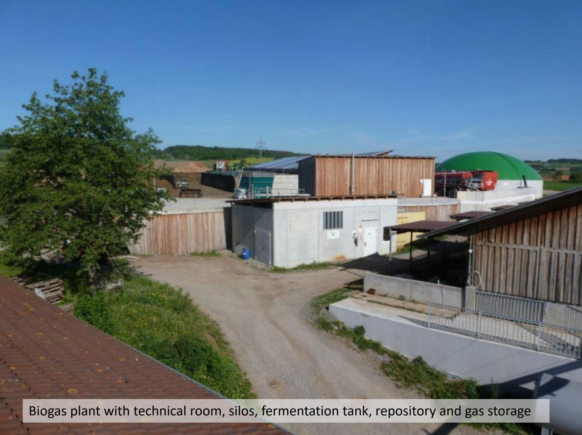
Biogas plant with technical room, silos, fermentation tank, repository and gas storage
